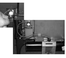
**14)** Connect fan ground wire to lug nut at base of unit.
